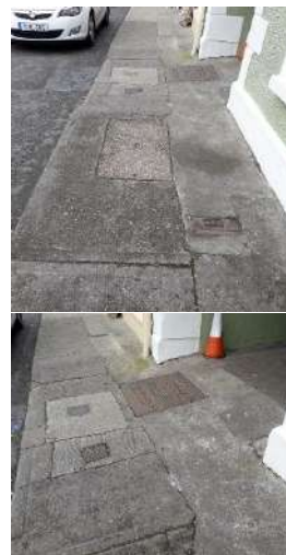
Figs 59 & 60 – concrete pavements with services
