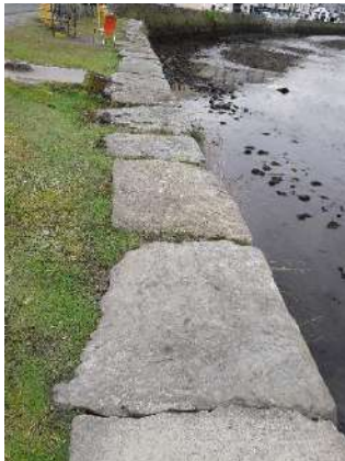
Figure 1 – Cover: Quayside wall parapet stones & cast iron crane base
