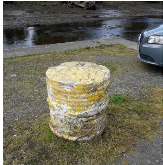
Fig 15 – concrete mooring bollard
