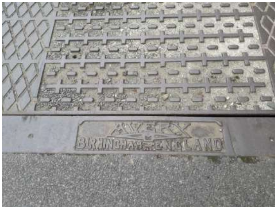
Fig 25 – detail on weighbridge in public road
