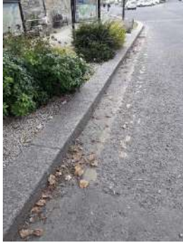
Figs 61 & 62 – previous pavement upgrades comprising Liscannor stone slabs and granite kerbs
