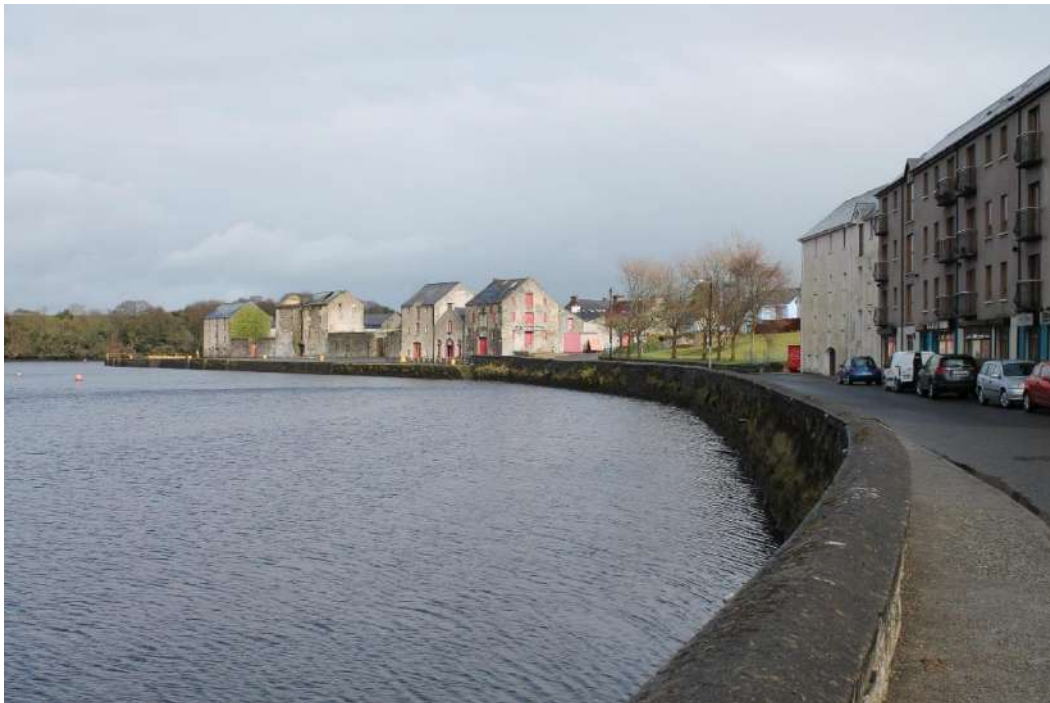
Figure 6 – looking east along the Shore Road towards the quay, warehouses and Ramelton Castle Site
