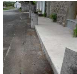
Fig 17 – new concrete pavement
