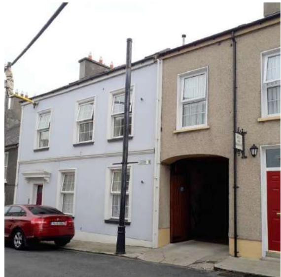
Fig 54 – cast iron sewer vent
