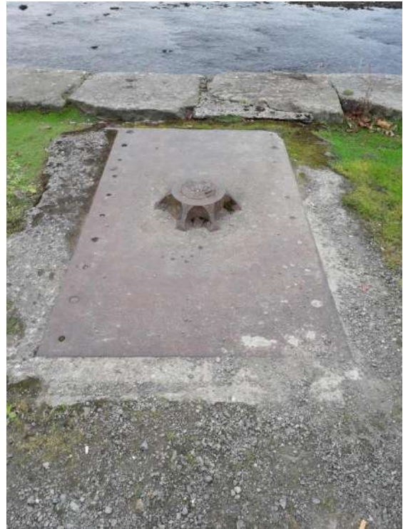
Fig 21 – base of former crane
