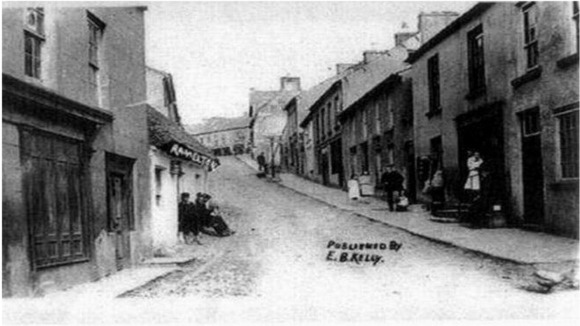
Figure 48 – view along Bridge Street towards the Market Cross from Gamble’s Square. Source Ramelton.net
