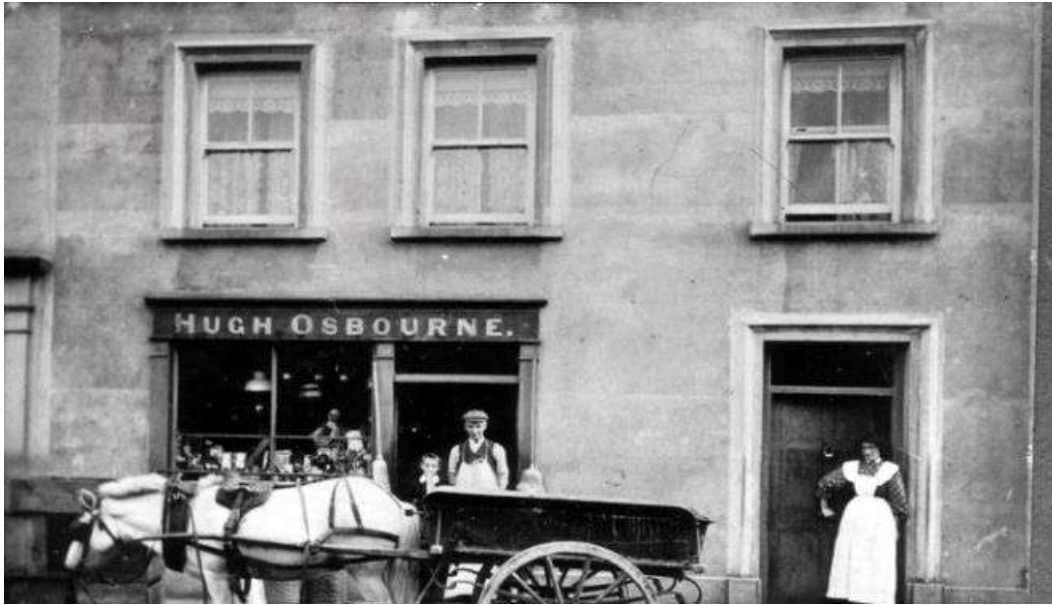
Figure 44 – former commercial premises at the east end of the Mall adjacent to the Tank Brae. Source ramelton.net
