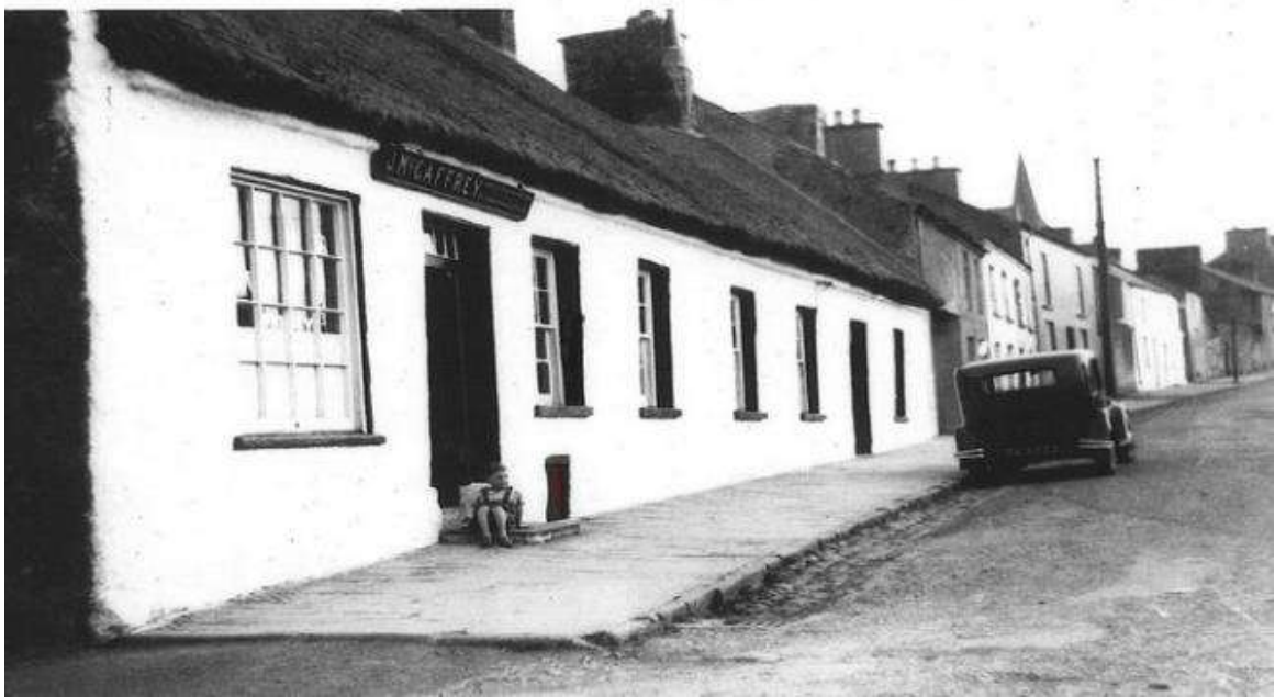
Figure 53 – thatched buildings on Castle Street. Source Ramelton.net
