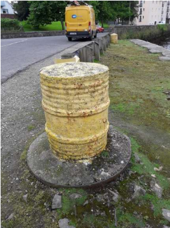
Fig 23 – concrete mooring bollard
