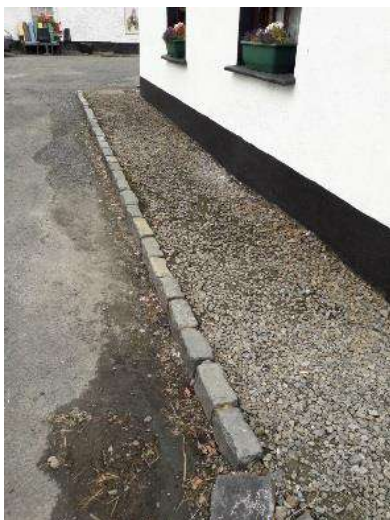
Fig 30 – stone blocks forming kerbline
