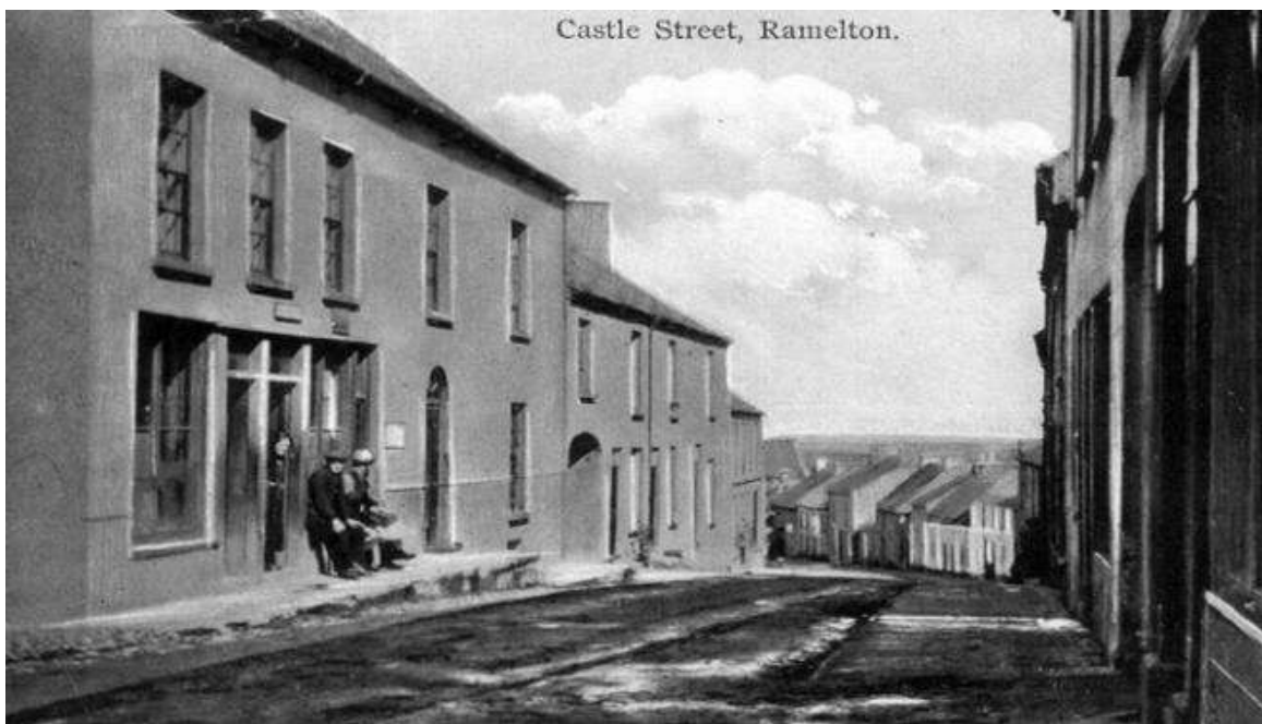
Figure 51 – the building on the left in Castle Street had been abandoned and in a semi-derelict condition for more than a decade. The façade has been recently restored as part of an Historic Towns Initiative Project Source: Ramelton.net
