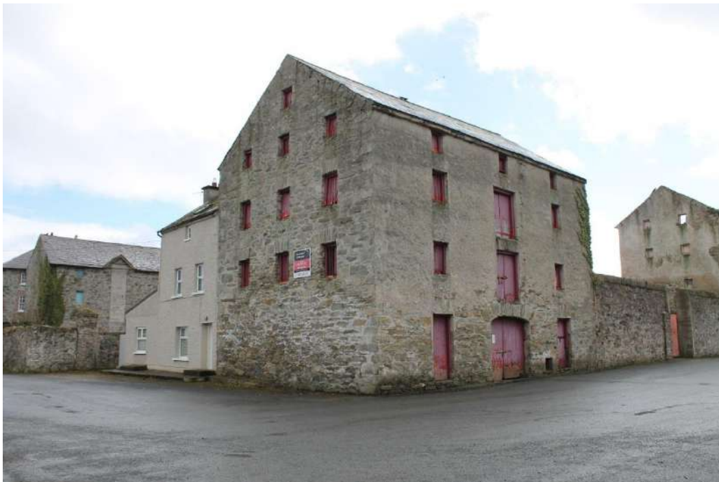
Figure 18 – quayside warehouse prior to recent conversion to two dwelling houses
