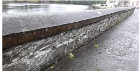
Fig 73 – stone wall with concrete coping
