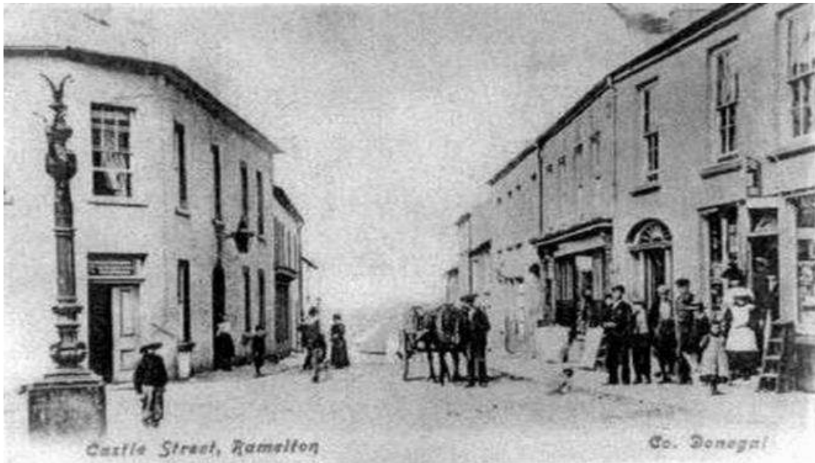
Figure 50 – commercial premises adjacent to the Market Cross. Source Ramelton.net
