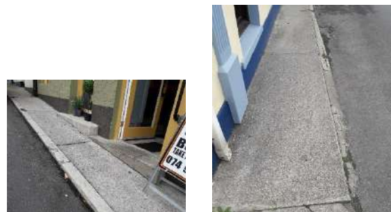
Figs 44 & 48 – generally concrete pavements
