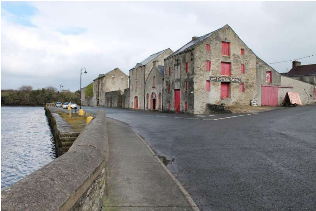
Figure 15 – view along the Quayside looking east
