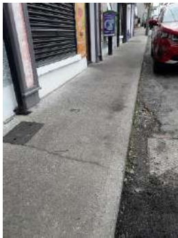
Fig 36 – generally in-situ concrete pavements
