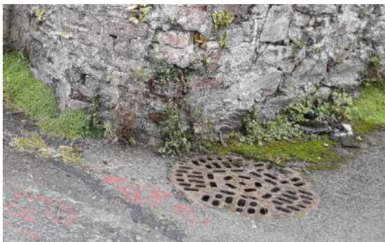
Fig 69 – grating at corner of steps above
